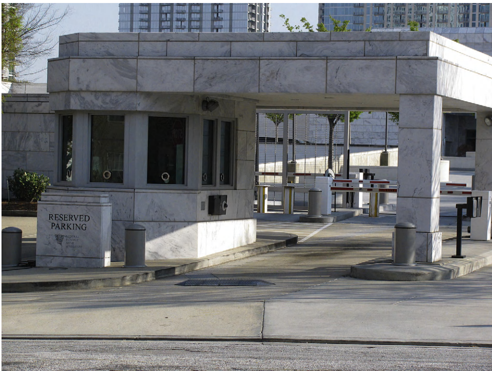
FIGURE 8-13 Access controls at a parking lot.
