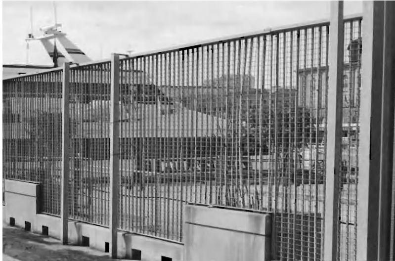
FIGURE 8-4 Anticlimb fence with vulnerability.
