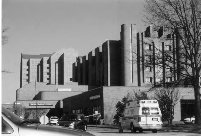
FIGURE 17-7 Healthcare institutions play a critical role in mitigating and recovering from the effects of natural disasters or deliberate attacks on the homeland. Physical damage to these facilities or disruption of their operations could prevent a full, effective response and exacerbate the outcome of an emergency.
