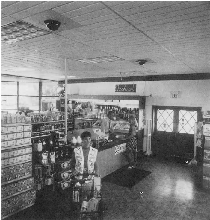
FIGURE 17-2 Checkout counter, CCTV camera domes, and electric article surveillance (EAS) system (portals at exit). Courtesy: Sensormatic, Inc.
