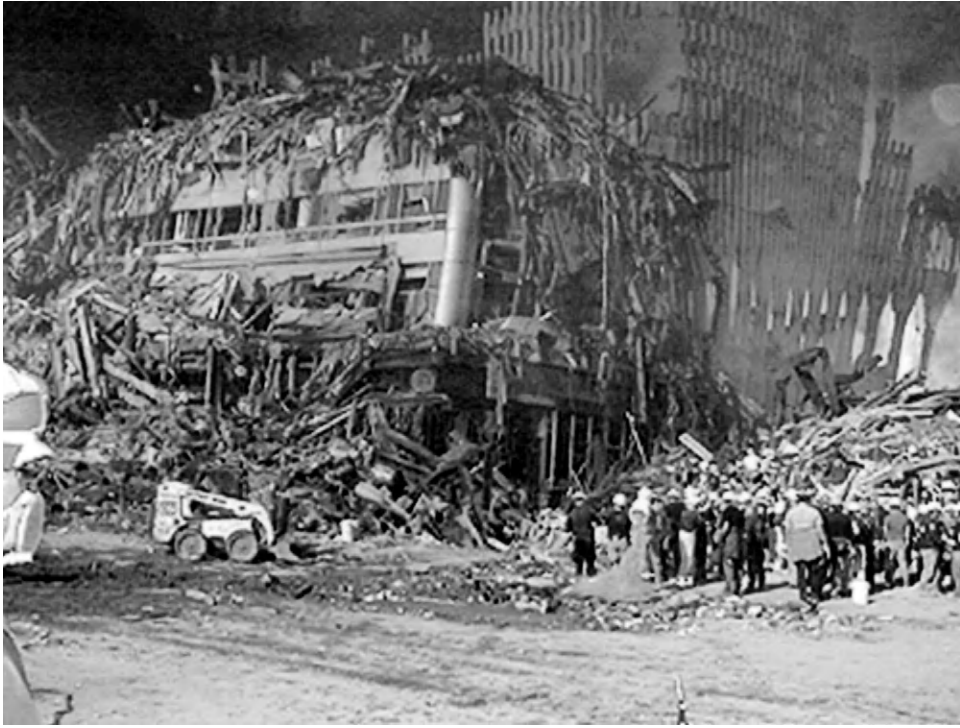
FIGURE 15-2 Destruction of the World Trade Center in New York City following the September 11, 2001 terrorist attack.
