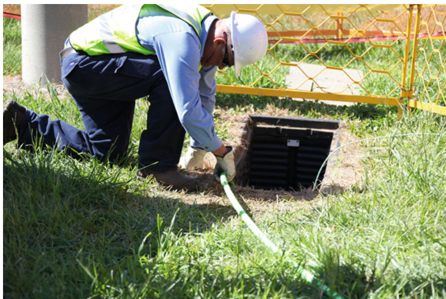
Optic fibre being installed underground. Source: Copyright © 2013 NBN Co Limited. All rights reserved 104
